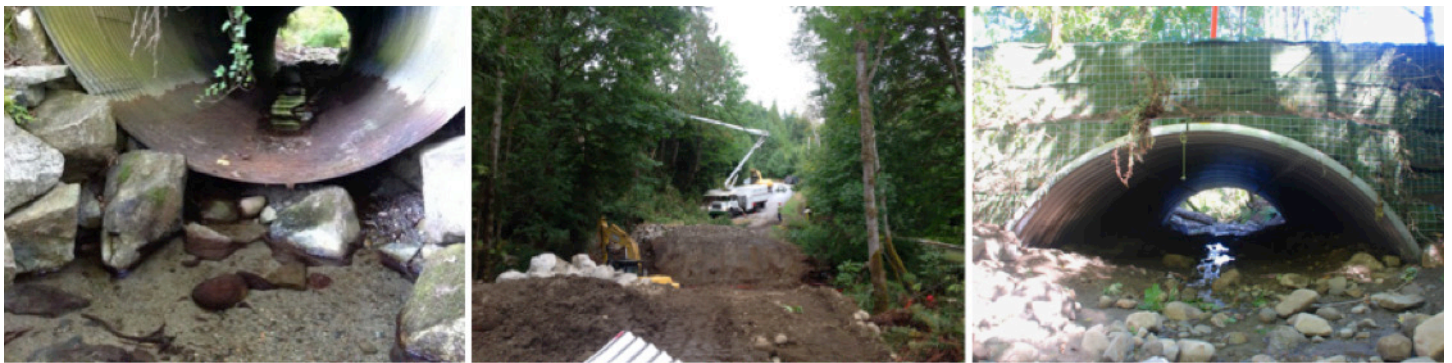
Spot the difference! Basil Creek culvert before, during.....and after!
